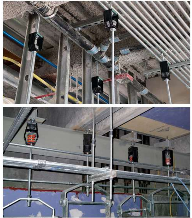
Fig. 2. Spring Hanger Used for Vibration Isolation and Thermal Expansion Accommodation In Industrial Piping Systems.
